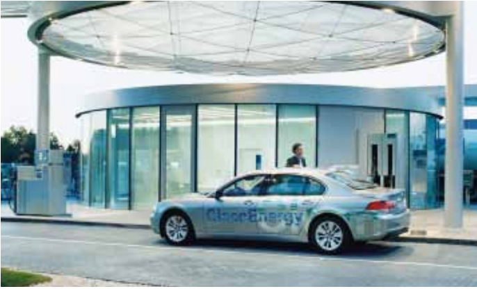
Linde hydrogen filling station in Unterschleissheim, Germany.
